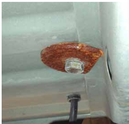
Figure 20. Load-spreading washer located under vehicle bed
