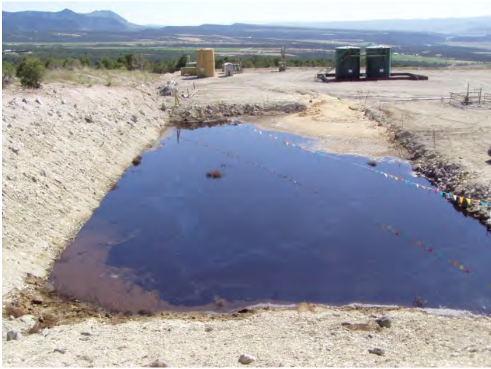
Figure 3. Reserve pit at a completed well site near Parachute, Colorado. (USFWS Photo by P. Ramirez)
