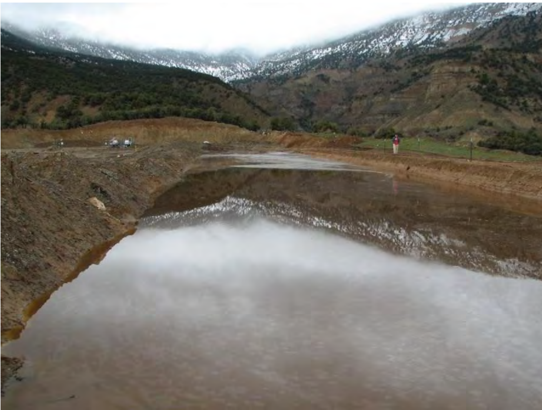
Figure 8. Trench used for burial of drill cuttings from closed-loop drilling. Sheens are visible on the water surface. (USFWS Photo by P. Ramirez)
