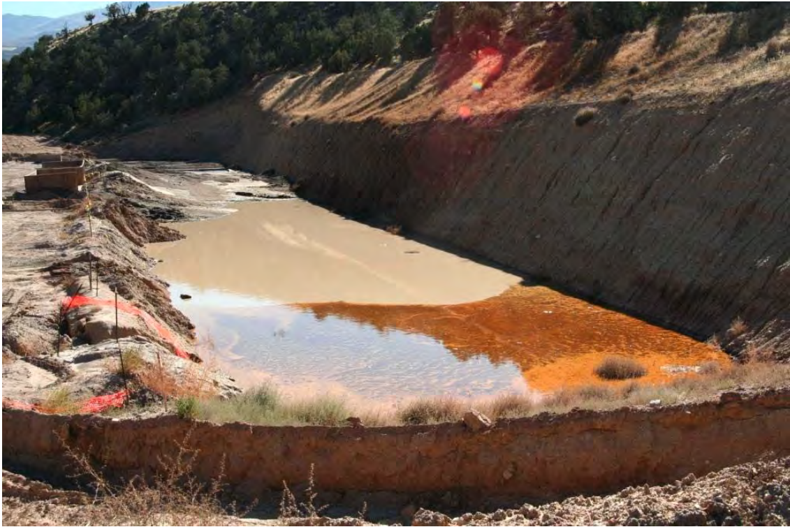
Figure 9. Ponding of snowmelt and rainfall in trench used for the disposal of drill cuttings from closed-loop (pitless) drilling system.
