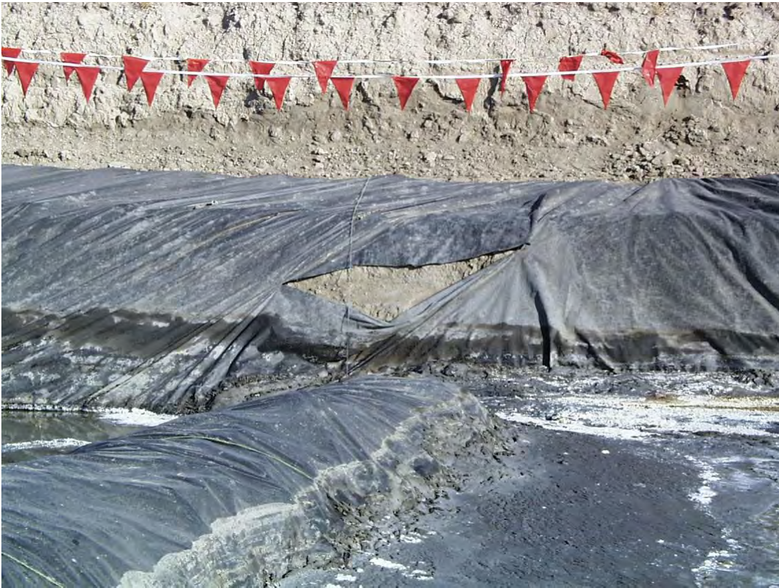
Figure 6. Reserve pit with torn synthetic liner. (USFWS Photo by P. Ramirez)
