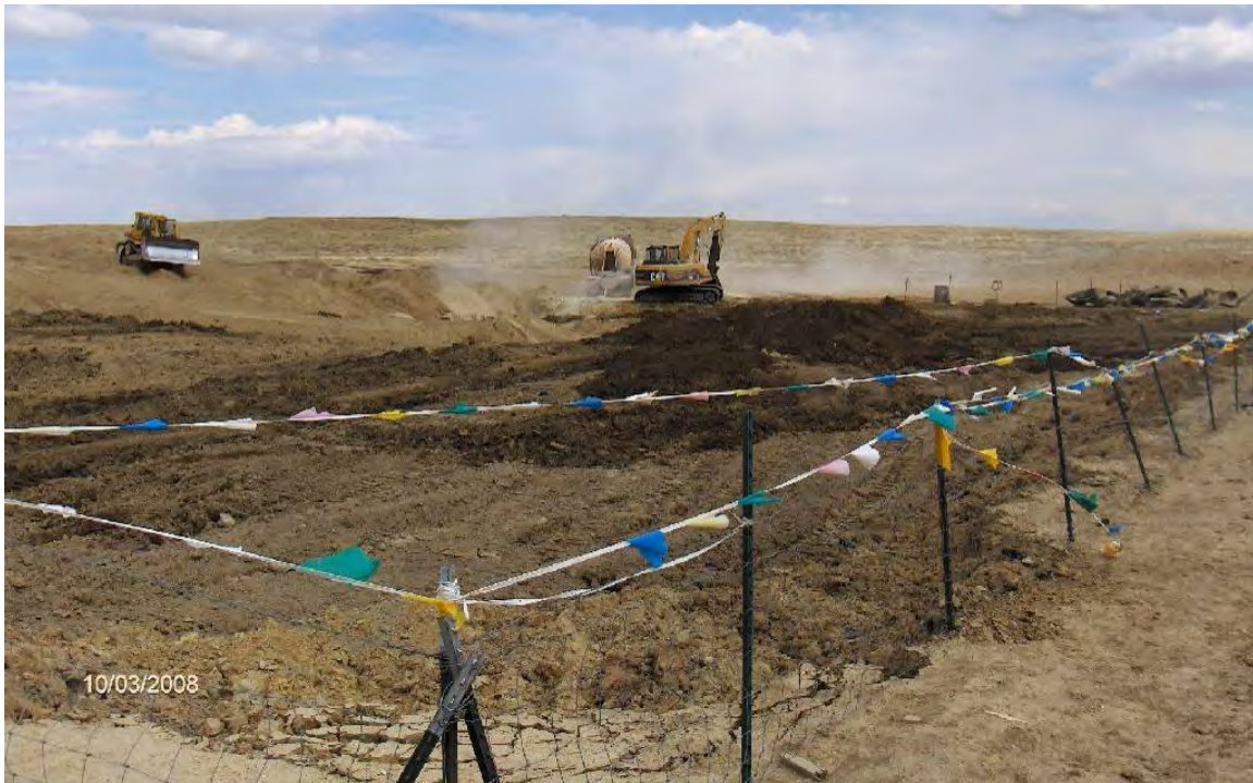
Figure 5. On-site burial of reserve pit wastes, Carbon County, Wyoming.
