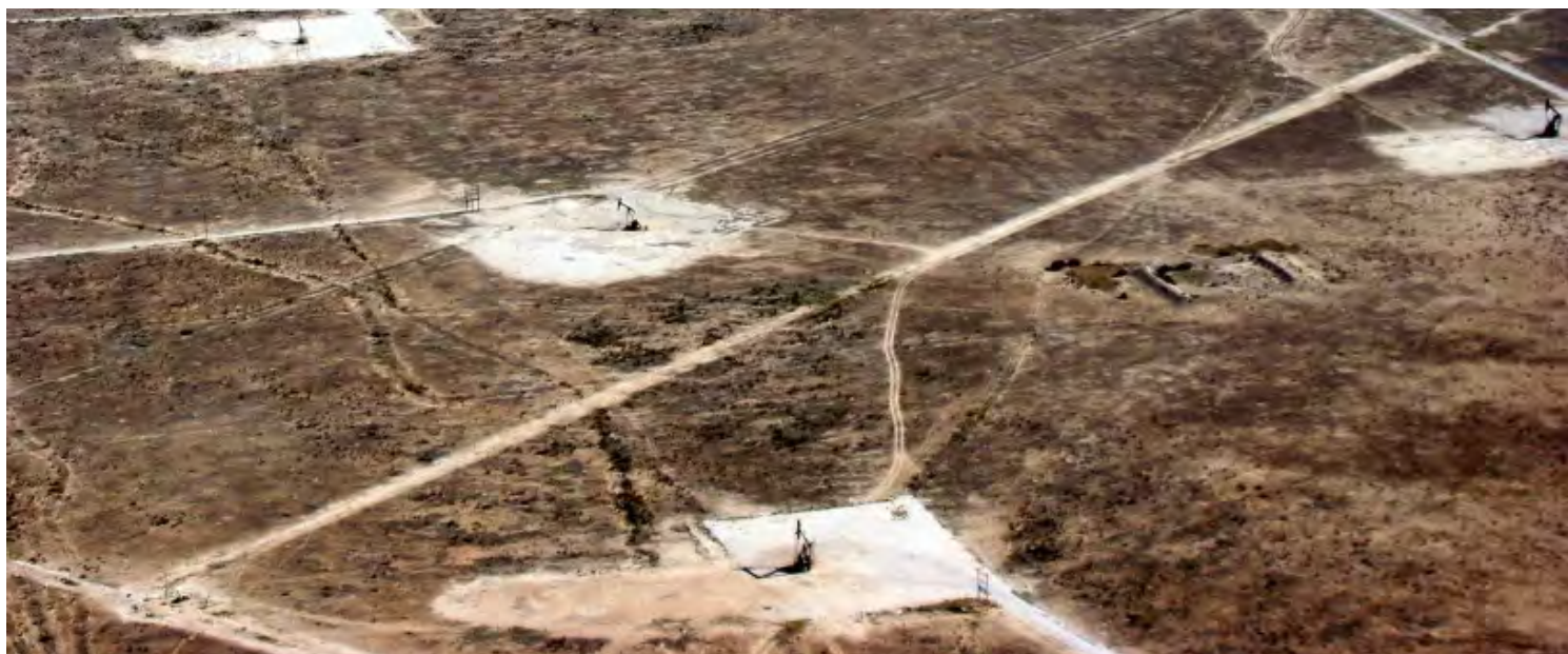
Aerial view of oil and gas infrastructure in the western Permian Basin of New Mexico.
