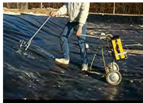
(b) Ultrasonic field monitoring
