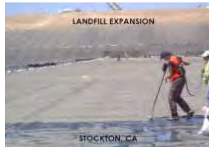
(c) Soil covering geomembrane
