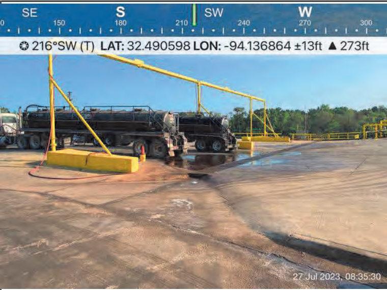
Vacuum trucks were unloading saltwater at the new unpermitted pit catch basin.
