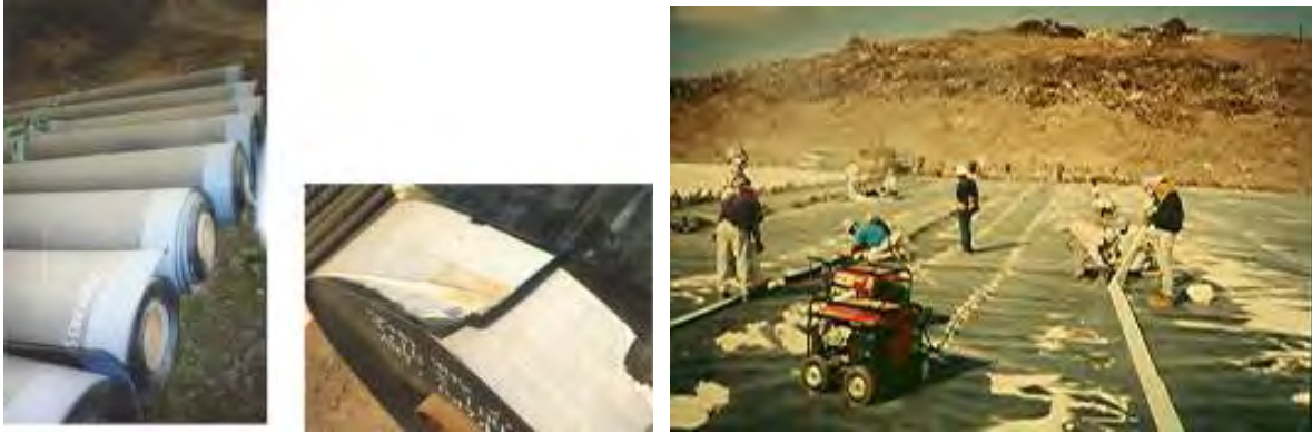
(c) Geomembranes with taped edges
