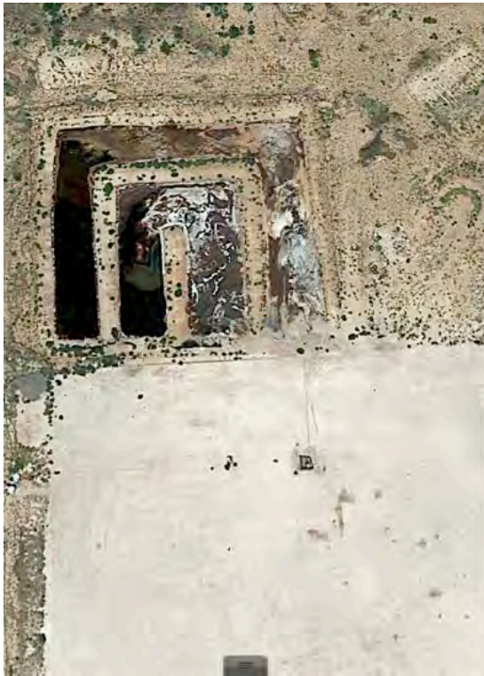
Figure 2. Reserve Pit (Permian Basin) with Extensive Chloride Impact
