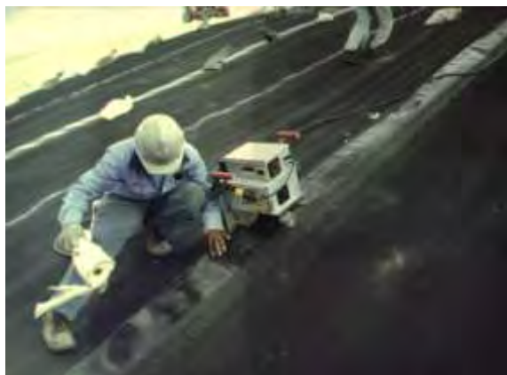
(b) Drying an area for seaming
