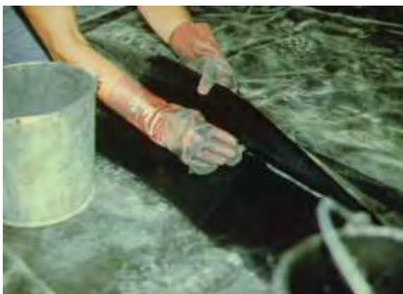
(a) Cleaning area for seaming
